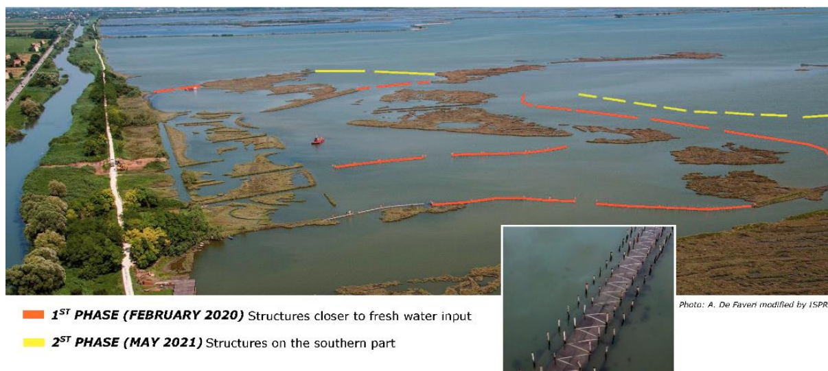
Figure 2. Aerial overview by drone of morphologic works
