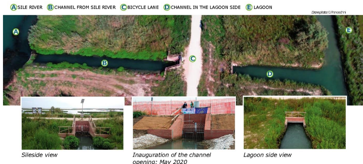
Figure 1. Aerial overview by drone of hydraulic works
