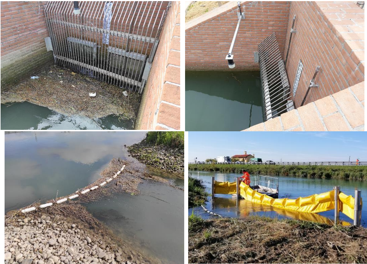
Figure 2. Photographs of some maintenance interventions near the hydraulic works.
