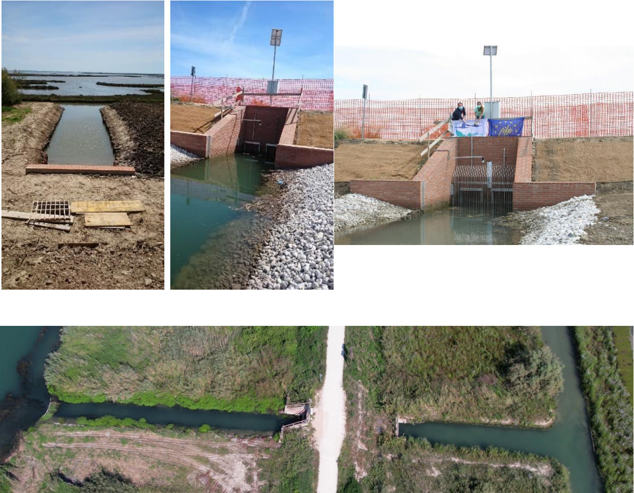
Figure 1. Photographs of the realization process of the hydraulic work.
